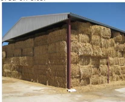
Hay storage in open-sided shed
